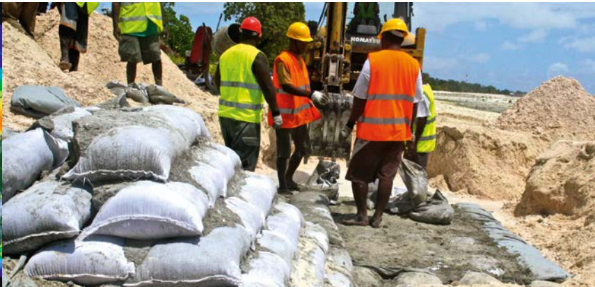
Constructing seawalls, Tuvalu
