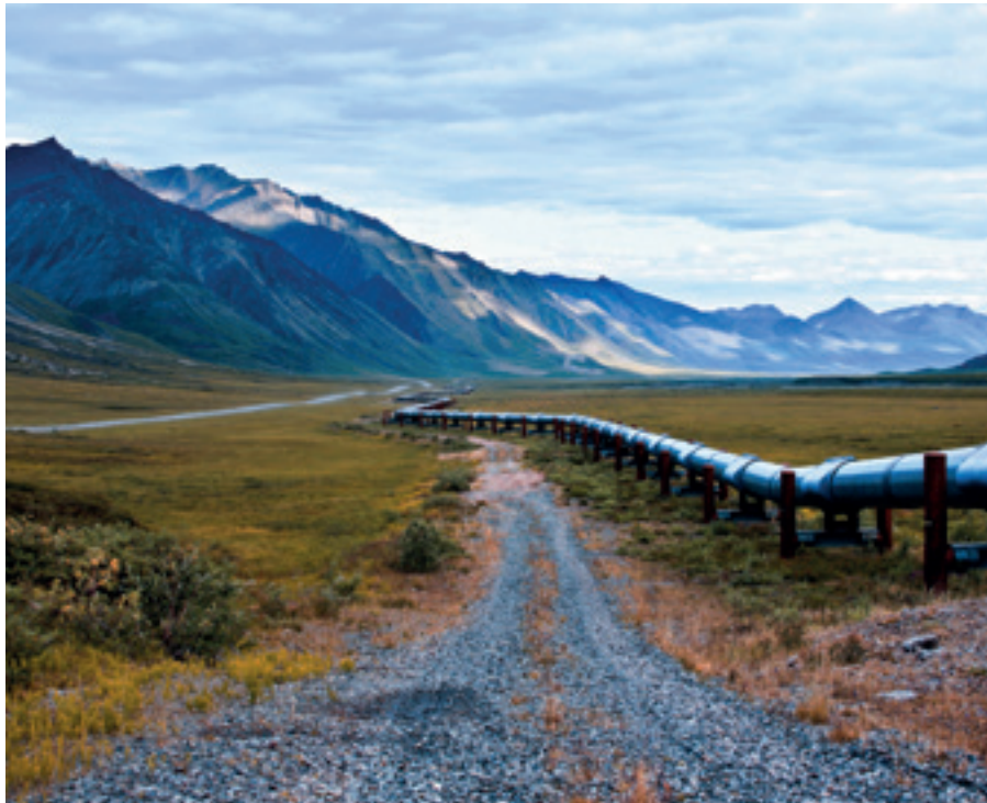
NORTH SLOPE PIPELINE, ALASKA ©iStock / Kyletperry
