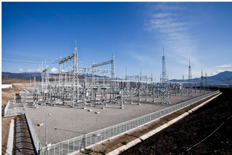
Back to Back Station in Akhaltsikhe, © KfW Image Archive/Rendel Freude
