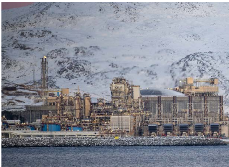
Melkøya gas complex near the town of Hammerfest
